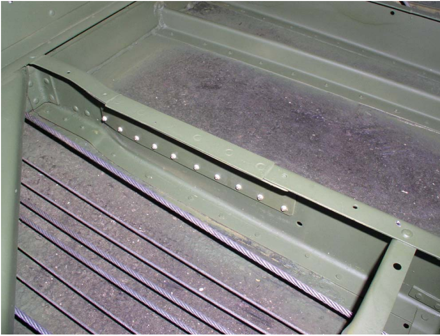
Completed floor structure repair.
