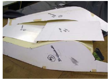
Fabricating patterns of the many seat panels.
