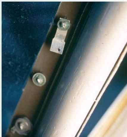
(5) Direct structural mounting method showing 1/4" holes drilled near the window's edge. Mounting hardware and sealer can also be seen in this photo.
