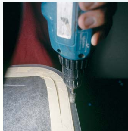
Rotary file being used to mill the standing edge of a milled-edge enhanced-thickness window.
