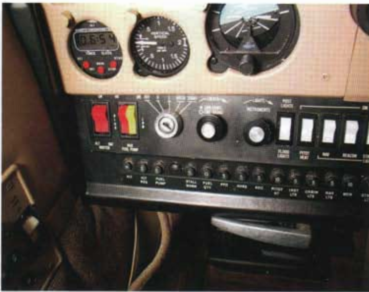
Repaired, re-painted and placarded sub-panel with removable circuit breaker placard strip.
