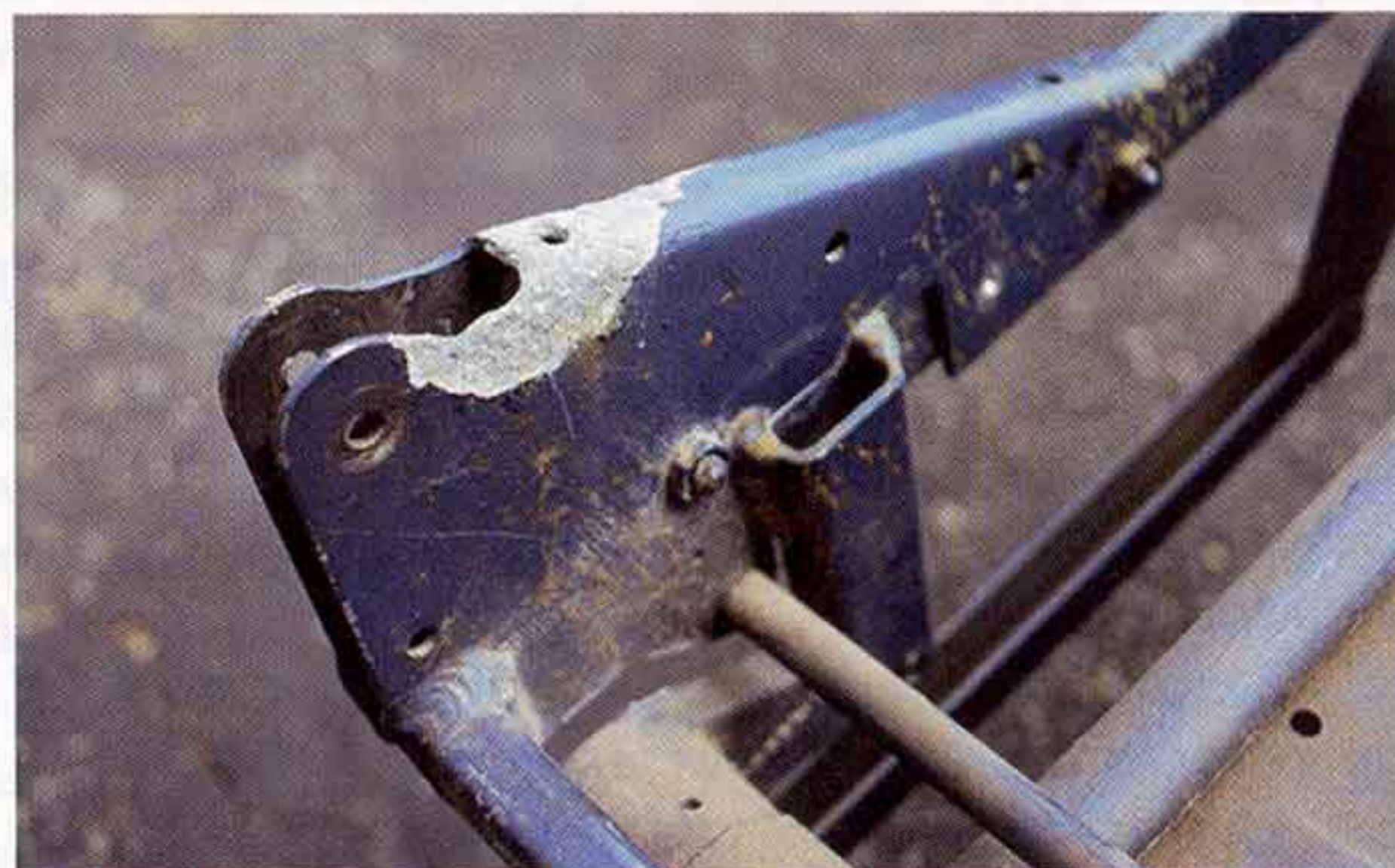
After-market flame treatments for upholstery materials are likely to cause corrosion, as in the photo above.
