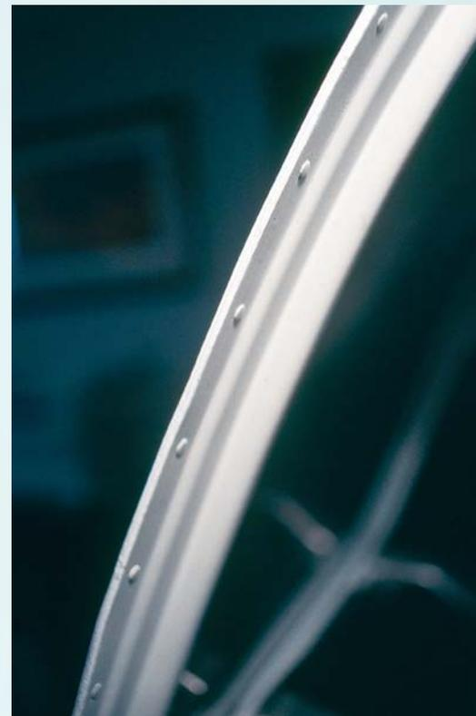
(2) End view of the center-opening window frame showing the 3/32" rivets used to fasten the inner and outer frame sections together.
