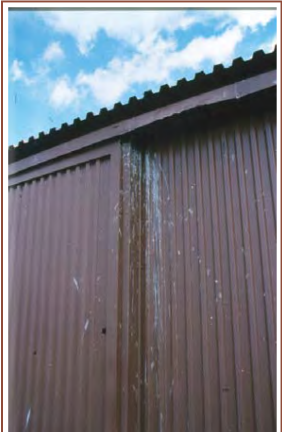
Bird droppings are signs of a serious bird problem in this hangar.
