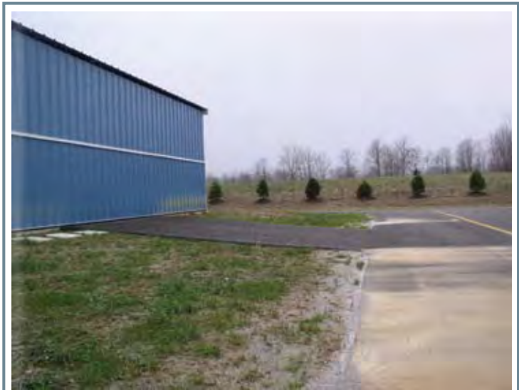
Sloping ramp indicates the hangar is definitely above grade.
