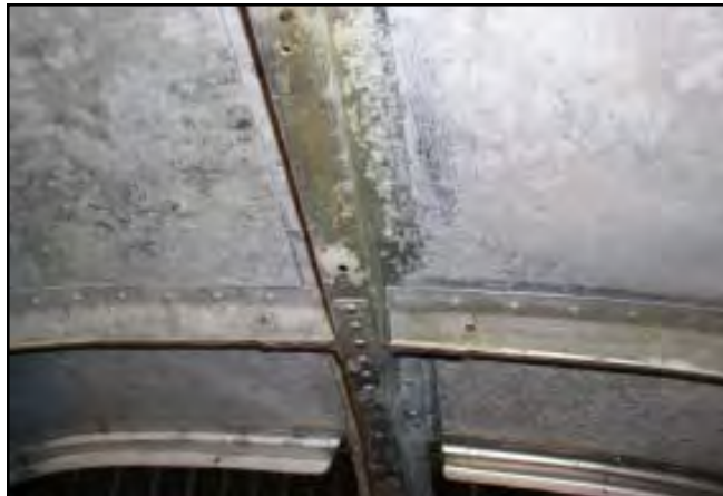
Typical corrosion found under the aft headliner of a 1974 172.
