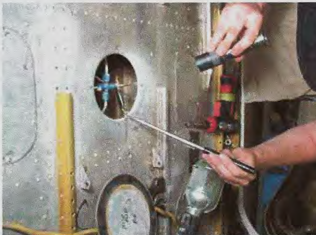
Using a bright flash light and an inspection mirror for the inspection in all the hard to see places
