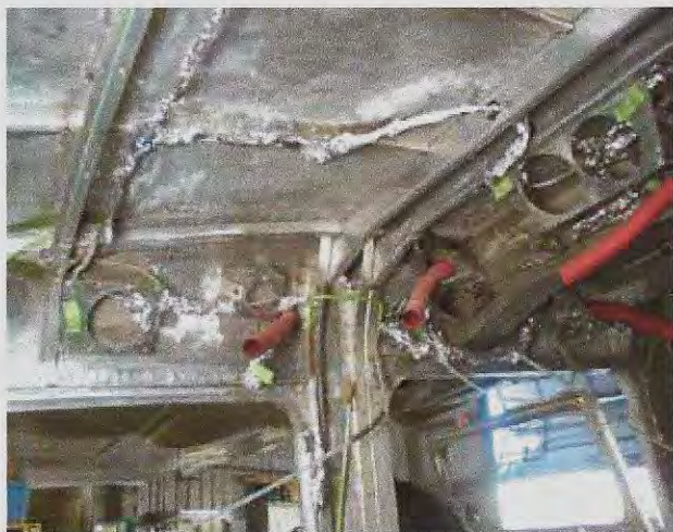
Thoroughly cleaned cabin ready for final solvent wipe down
