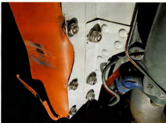
A cracked corner, repaired with rivets and a doubler scarf patch.
