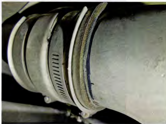
A black line drawn with a marker helps identify a loose turbo system coupling hose.
