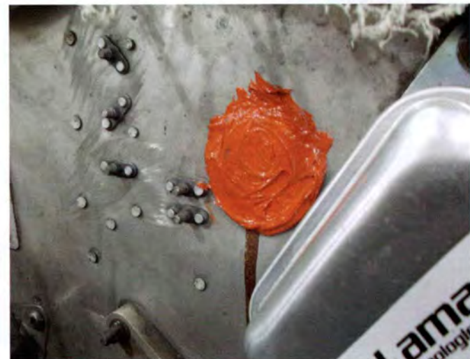
Sloppy use of high-temperature silicone covering an unused, riveted-in-place firewall patch.
