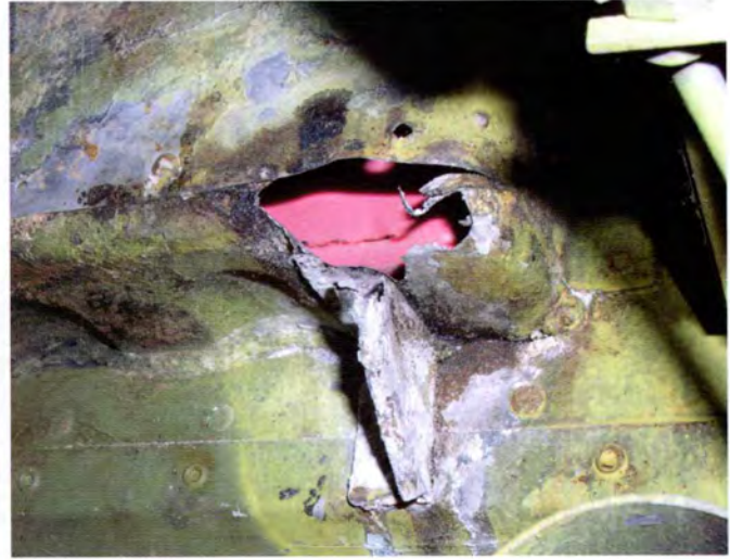
Severe battery acid damage in the lower corner of an aluminum battery box.
