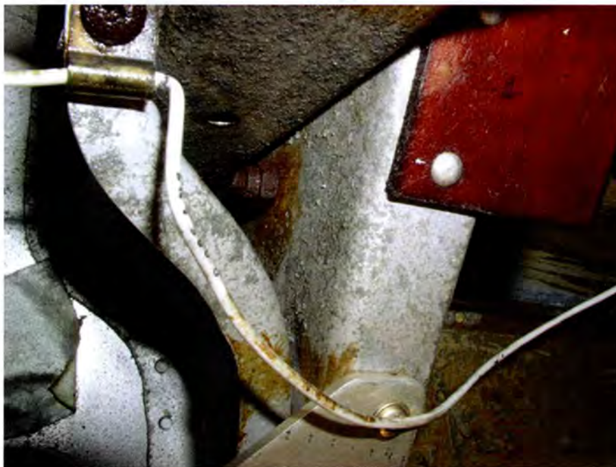
Severely corroded aft wing spar attach point in an airplane represented to the buyer as being almost corrosion-free.
