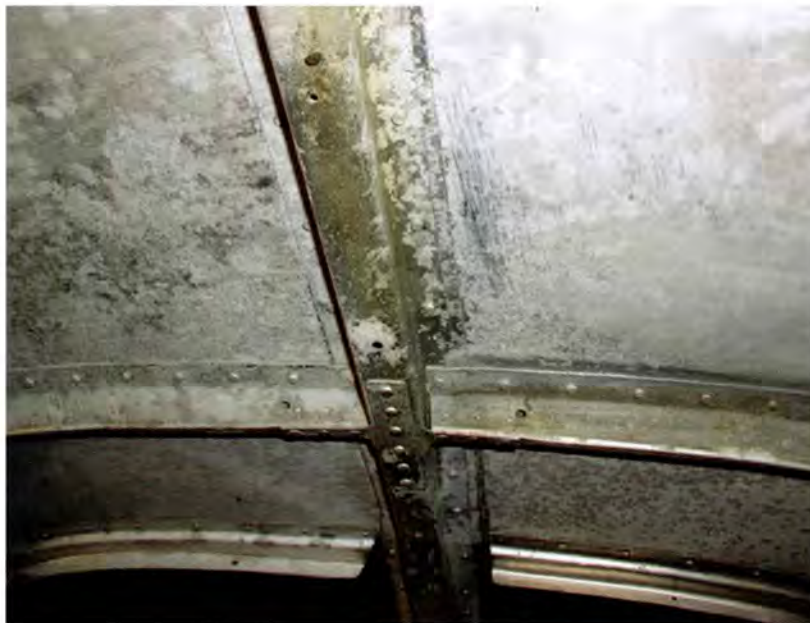
Surface corrosion on an upper cabin skin.
